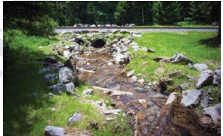
under the track that connects Spruce to Cass Scenic Railroad State Park. Rather than remove the culverts, biologists planned to install a culvert liner with prefabricated baffles that would create step pools in the culvert. These pools could be easily navigated by fish moving upstream.
